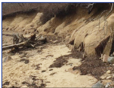
Outer Harbor eroded bank just past Sailing Class Beach
