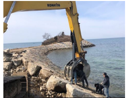
The team from C. F. Briggs Marine Construction places one of the large armor stones on the last 118 feet.
