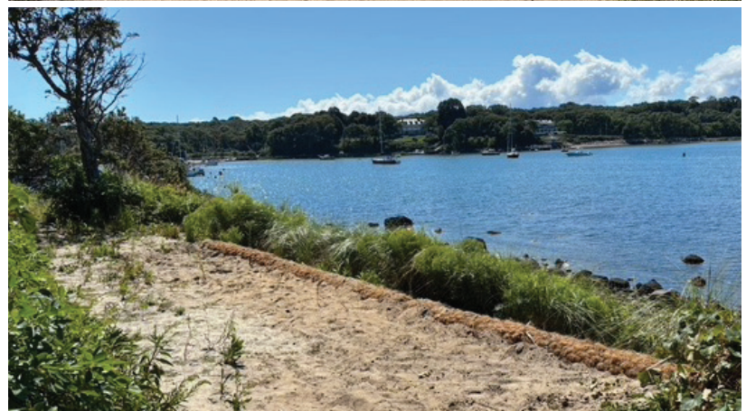
New coir log reinforcement at the outer harbor bank will limit erosion from rain runoff.
